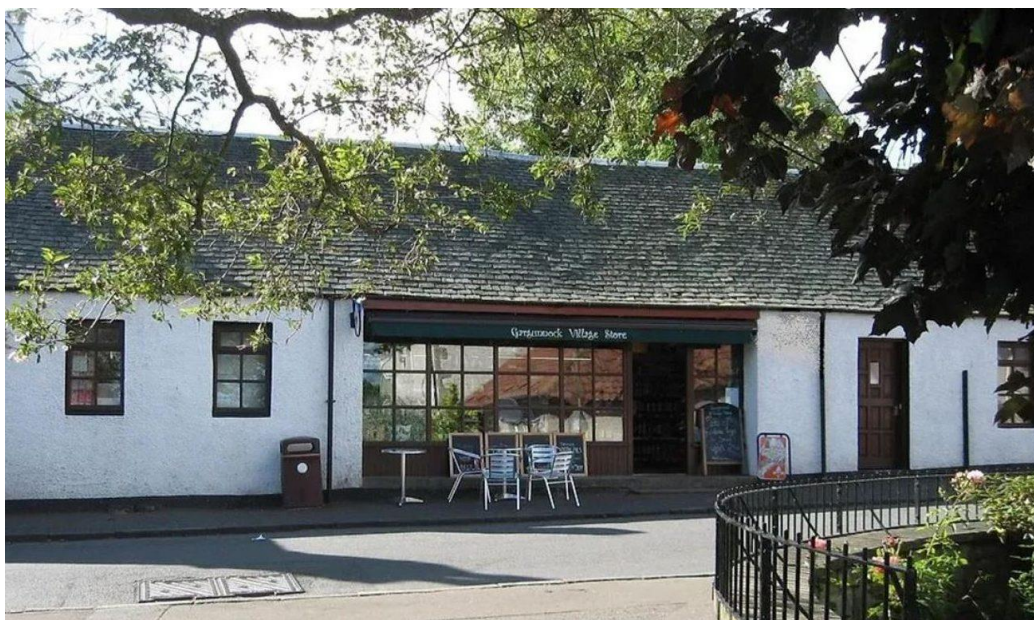
Figure 4: Gargunnoch Community Shop (Prior to Renovation)
